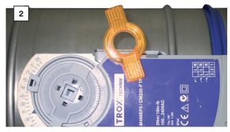
Place the magnet on the point indicated with "magnetic gear release". The gearbox is now disengaged and the actuator can be moved. 1
